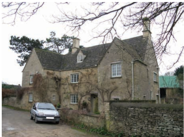
Mill House, Mill End
