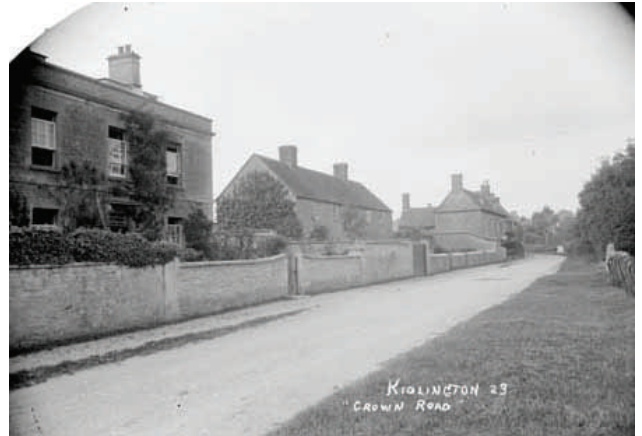
Limestone walls continued from Exeter House to the smaller cottages
