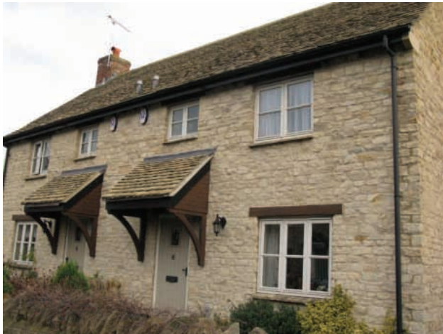
Well-designed and maintained modern properties can fit well beside older ones when sympathetic measures are taken
