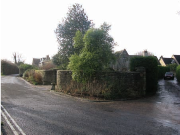
The curved wall of no. 42 at junction
