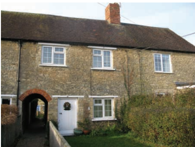
The brick archway with a glimpsed view of the cottages beyond
