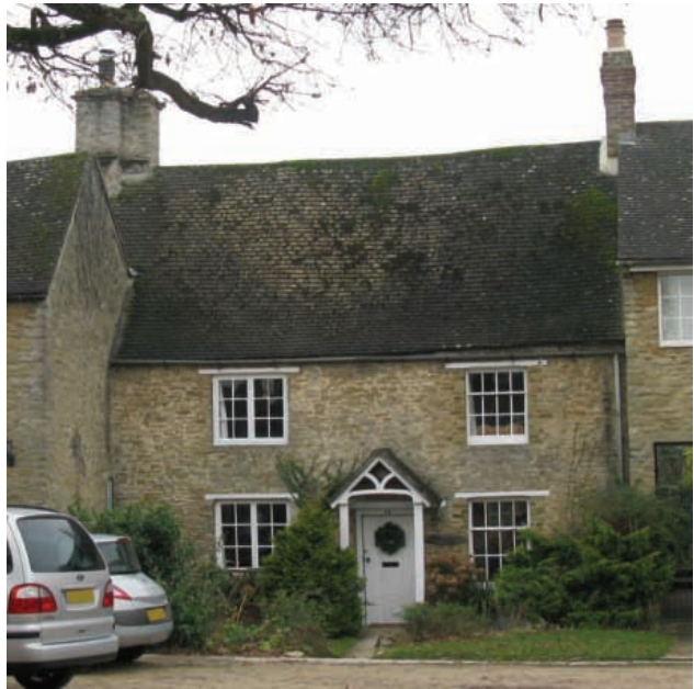
Bellhangers, 64 Mill Street
