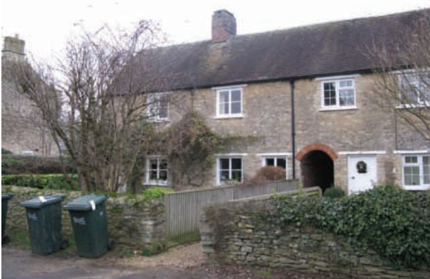
Nos. 30 and 32 retain their stone boundary walls
