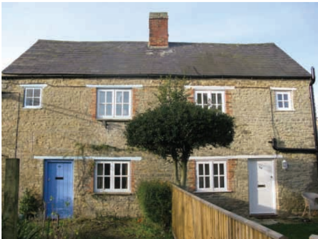
36-38 Crown Road: hidden gems behind the main terrace
